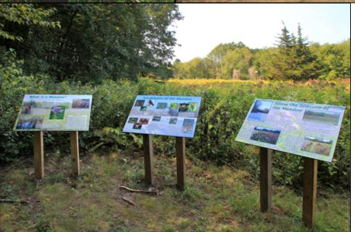
QTY SIZE DESCRIPTION PRICE / RATE TOTAL 2 22" x 46" MANUFACTURE NEW SIGNAGE Panel Fabrication: 1/2" High Pressure Laminate 2 24" x 48" MANUFACTURE - SIGN STAND Fabrication: 1/4" aluminum plate, primed and painted attached at an angle to (2) 4" x 4" aluminum square tubes, primed and painted for direct embedment into concrete footing
